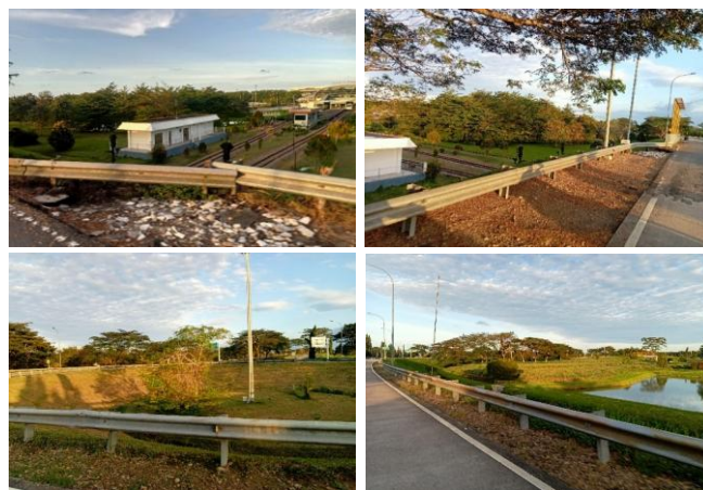
Figure 2 The area of Kualanamu Airport Access Road that has steep terrain
